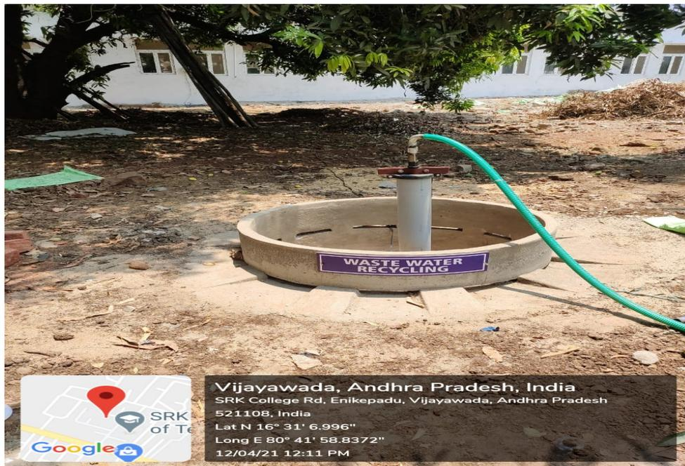
**Filtered water collected into a Bore well and lifted using 1 HP Pump**
